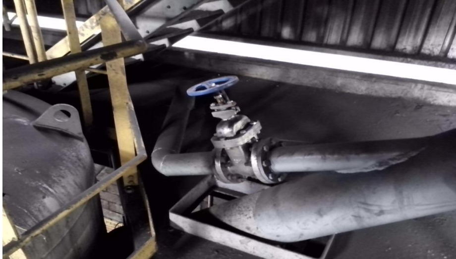
Gambar 4. Pipa Bypass 453-PF1
