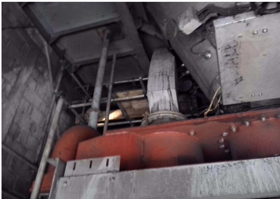
Gambar 5. Pipa Bypass 453-PF1
